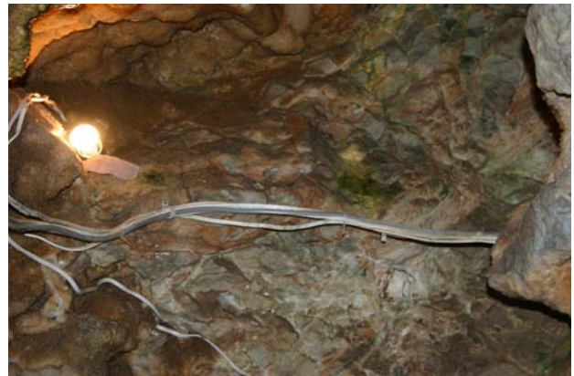
Exposed conduit in Wonderland Cave
